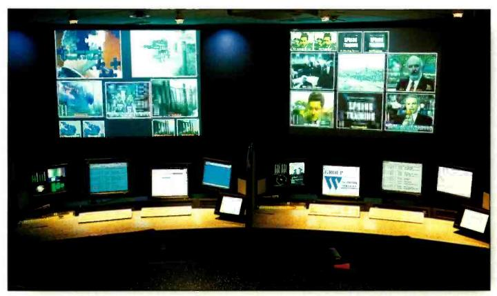
The master control facility at Harbor Plaza serves strictly as a monitoring station for automation systems in both facilities. Besides the monitors and projectors, there is no other electronic equipment in the control room.
