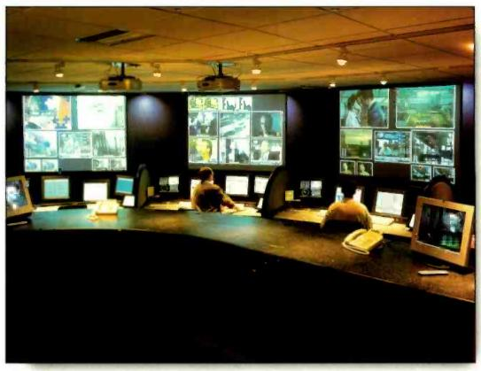
In GWNS' master control facility, five master control stations each handle four networks, monitoring four video images for each network's signal path.
